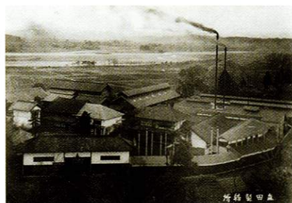
Fig.240 Complete view of the Morita Silk Mill (Taisho Period). The Tama River and the Okutama mountains appear behind the factory. In 1914(Taisho 3), the factory was powered by 2 steam engines, 16 hp and water 2hp.
