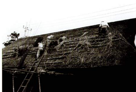
Fig.215 Thatch replacement (Ushihama, 1986 (Showa 61)).
