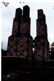
Fig.176 Nirayama reverberating furnace (Izunokuni City, Shizuoka Prefecture). Late in the Tokugawa shogunate cannon sizes increased so larger volumes of cast iron were required. The shogunate completed a reverberatory furnace, a Dutch designed metallurgical furnace, in 1856 (Ansei 3).
