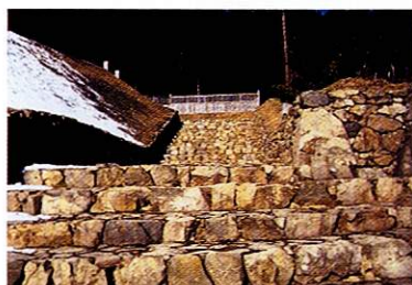
Fig.119 View from Hachioji Castle's main building toward its entrance.Route to the main building via detachable bridge, passage, stairs, and entrance. The outside slope is covered by the stone wall used as rampart.
